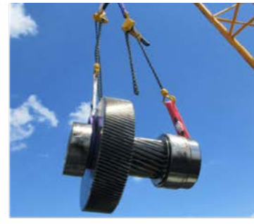
Picture 6. Damaged IMS removal.
